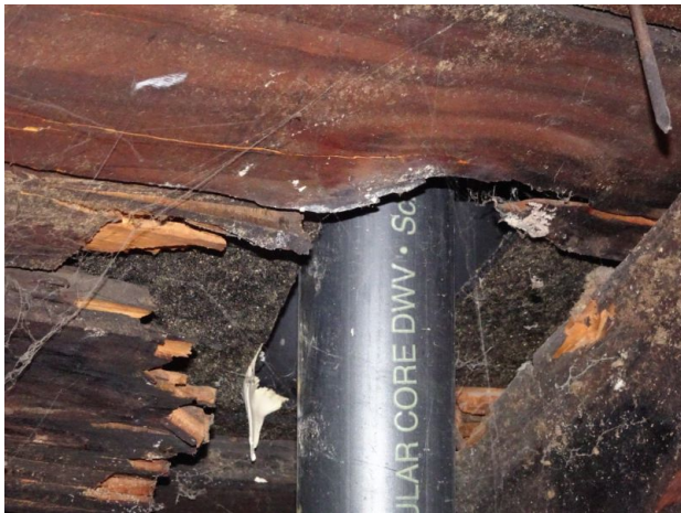
Bathroom vent not properly sealed. Wood sheathing damaged.
