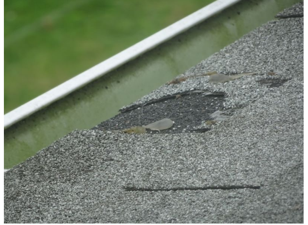
Broken shingle over side stairs.
