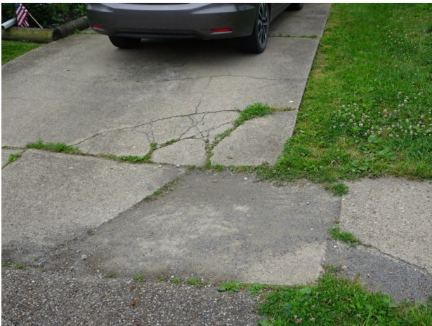
Driveway deteriorating.
