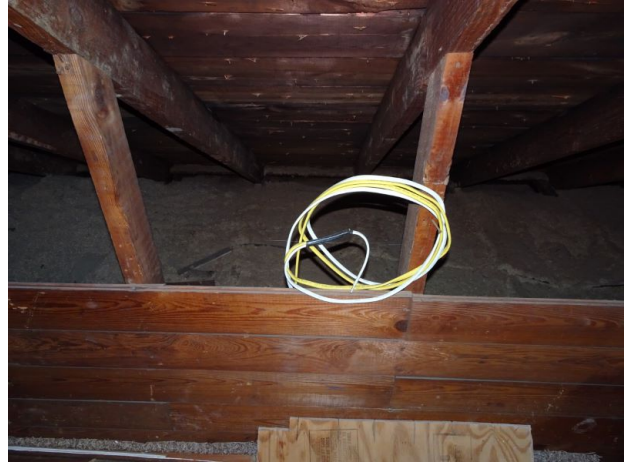
Exposed wiring.
