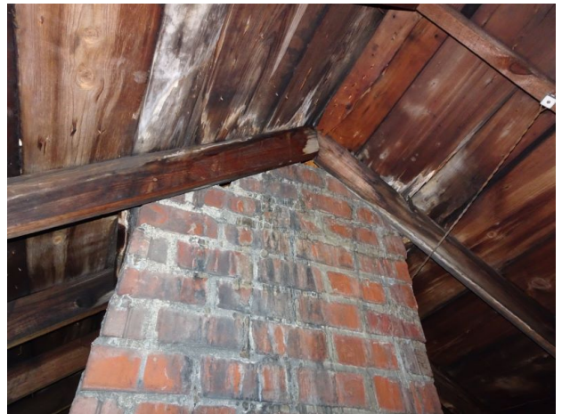
Old water damage.
