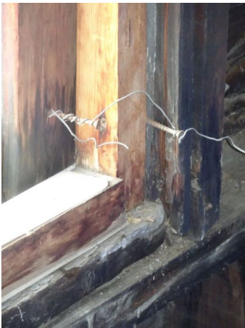
Back window fastened with screws and wire.
