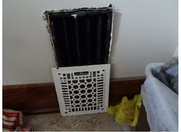
HVAC register cover unattached.
