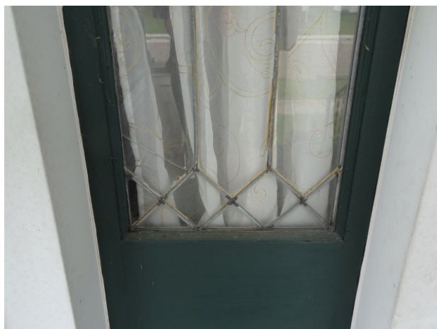
Entranceway cracked glass.
