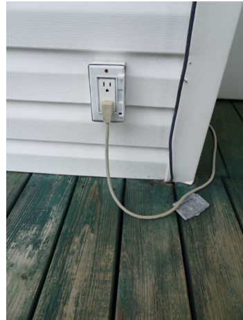
Broken outside outlet cover.
