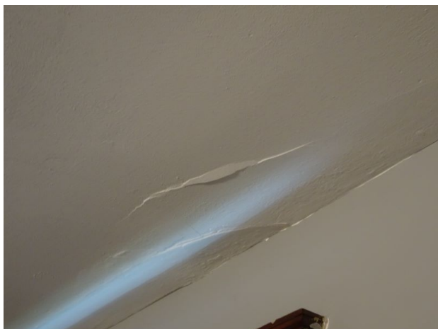
Front right bedroom ceiling bulging.
