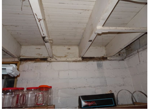
No insulation along rim joist.
