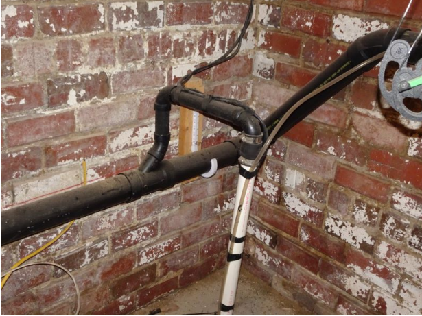
Sump pump connected to sanitary sewer line.
