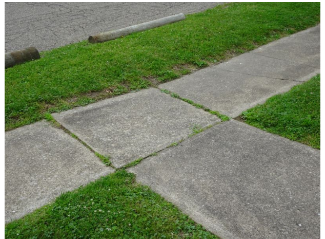
Sidewalk sinking.
