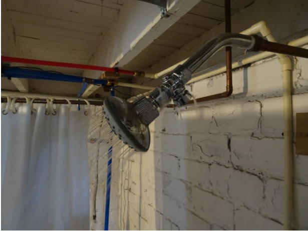
Basement shower head leaking at fitting.
