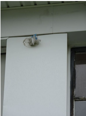
Missing outside light fixture.
