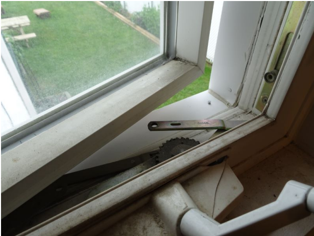
Window closer is broken.
