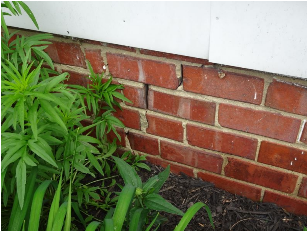
Settlement crack.
